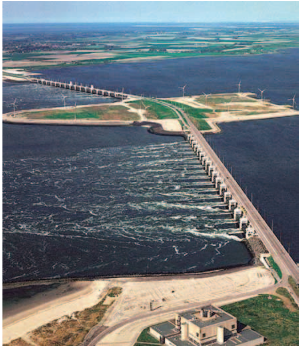
Figure A.47. Eastern Scheldt Storm Surge Barrier along the North Sea coast of the Netherlands, a seawall eight kilometres long. Its sixty-two openings are closed off with sliding barriers at high tide.
