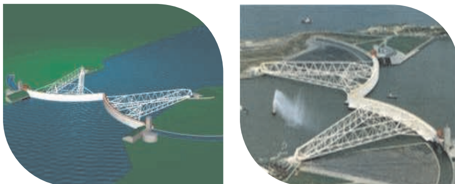
Figure D.7. A drawing and photograph of the waterway storm surge barrier in the closed position at Rotterdam in the Netherlands.
