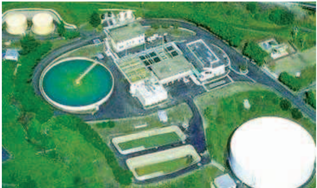
Figure 13.3. A 6-million gallon per day water treatment plant at San Luis Obispo, located about halfway between Los Angeles and San Francisco on the central coast of California.
