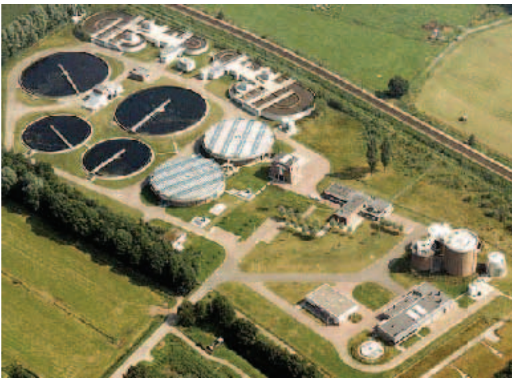
Figure 13.8. Wastewater treatment plant in Soest, the Netherlands (Waterschap Valleien Eem).
