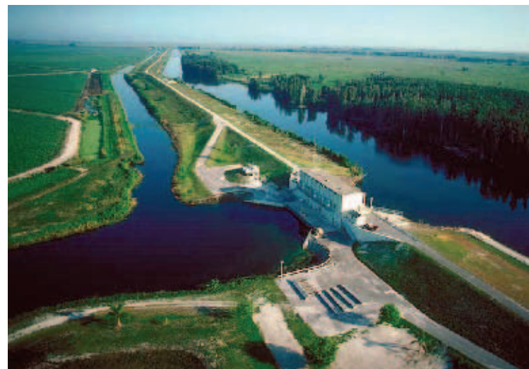
Figure 1.11. Pump station on a drainage canal in southern Florida (South Florida Water Management District).
