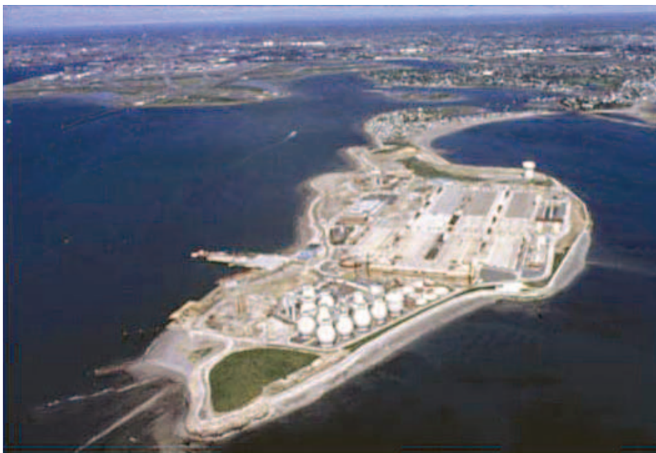
Figure A.44. Deer Island Sewage Treatment Plant in Boston Harbour treats and discharges an average daily flow of about 380 million gallons (1.43 million m 3 ) of wastewater. (With permission of Piping Resources Partnership of New England.)
